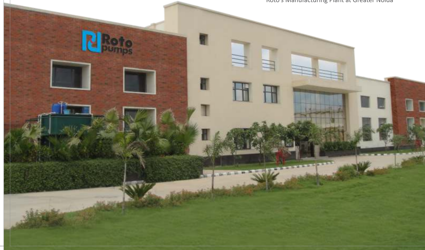
Roto's Manufacturing Plant at Greater Noida
